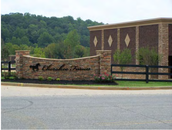
Brick and stone construction and signage
