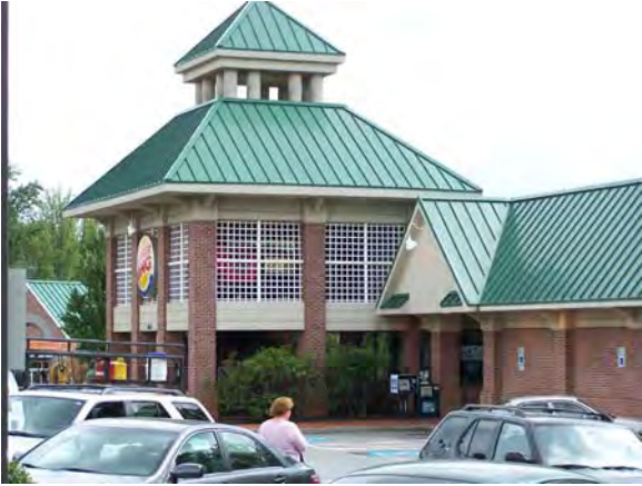
Architectural variation/features, brick construction
